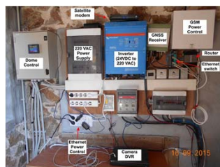
Transponder deployment at CDN1 site is complete. All instruments and devices are controlled remotely via satellite and 3G communication links.
