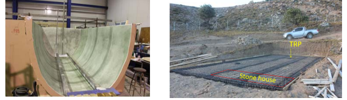
The transponder "igloo" roof (left) and current construction status (right)
